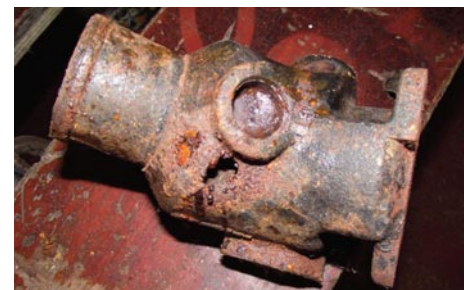
Volvo manifold Perforation of the cast iron manifold due to corrosive salts.
